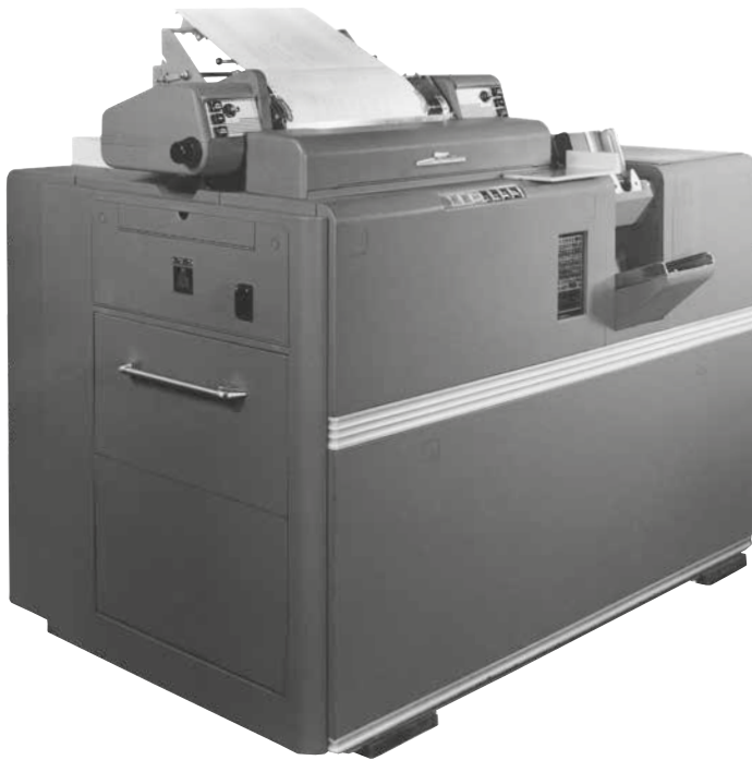
The tabulating machine IBM 421 was groundbreaking for the work of Allianz's punch card departments because it could write numbers and letters.
